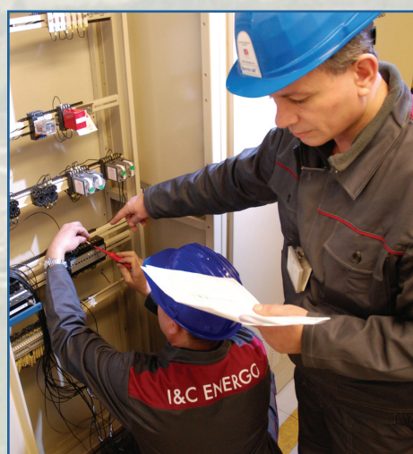
Installing relay wiring in a cabinet
