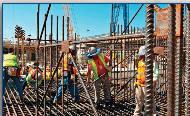
Construction of the turbine building for Vogtle Unit 3 in Georgia, USA
