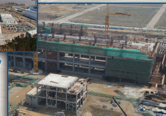
Construction of the conventional island for Haiyang Unit 2 in China
