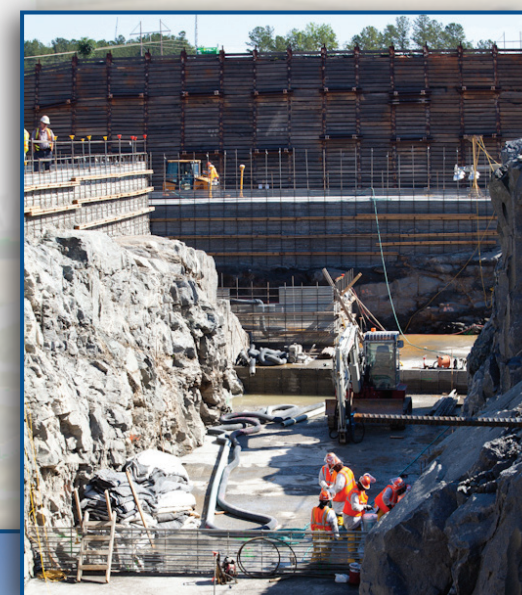
Excavation of the nuclear island for V.C. Summer Unit 2 in South Carolina, USA
