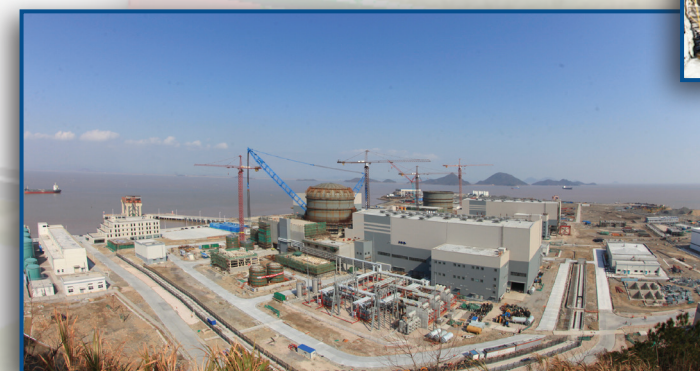
Overview of construction activities at the Sanmen site in China
