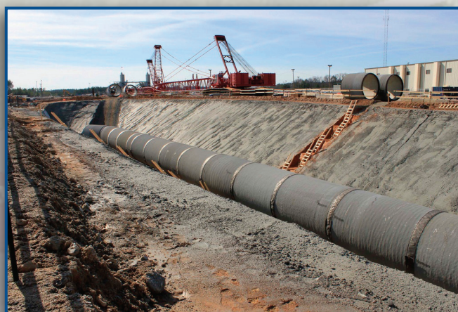
Installation of circulating water system piping for V.C. Summer Unit 2 in South Carolina, USA
